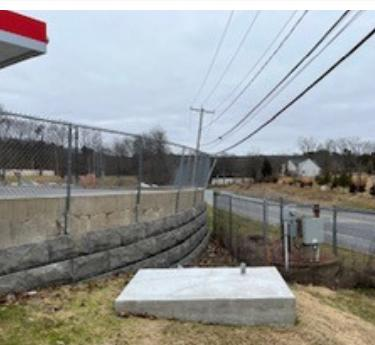
Concrete pads build by Public Works Department for new generators for pump stations.
